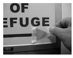
3C. Barely touch the adhesive side of the Arrowhead to the sign, and align the "stem" of the Arrowhead with the line (no overlap)
