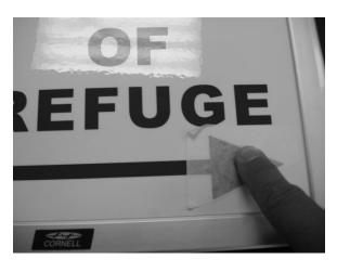
3D. Once properly aligned, smooth the arrowhead down. Gently squeeze-out any air bubbles.
