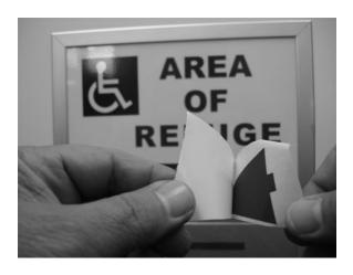
3B. Peel-off the backing (Keep translucent cover sheeting attached as shown – it provides a "handle" for alignment)
