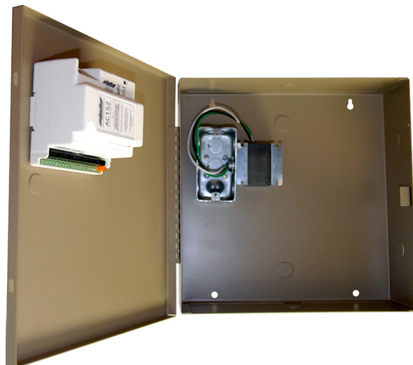
Figure 6 SS106 Transformer Installation
